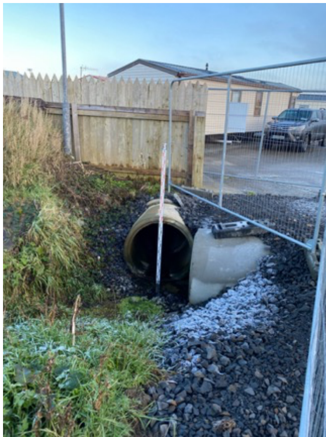
Figure 9 – Inlet to Culvert routed under Western Boundary of Caravan Park
